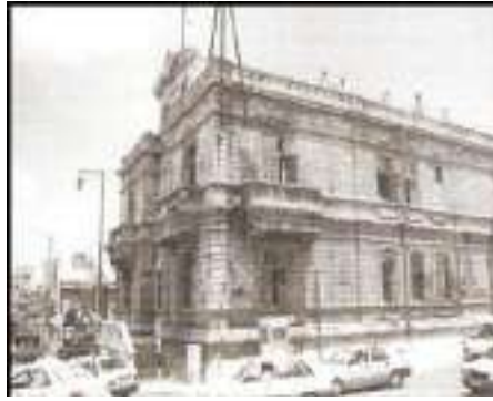
Figure (3-3) Old Municipal Building, Immigration and Passports Building, (حريثاني, 2006).
